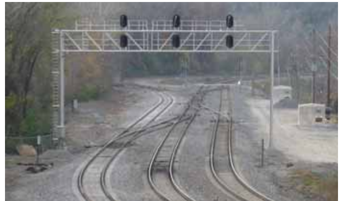
- BNSF Railway Sample universal crossover, at CP Congo on BNSF east of Kansas City, used by Amtrak's Southwest Chief . Trains traveling in either direction can move from any track to any other without backing up.
